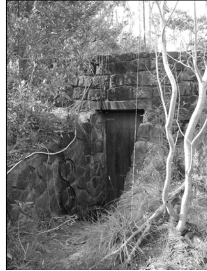
Figure 17. Mauna Loa Truck Trail Seismograph Vault LCS ID 058267, view to northeast.
