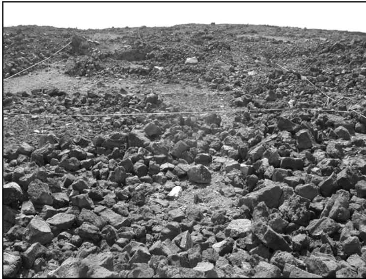
Figure 34. Site 50-10-50-5507, Features M-70, M-74, and M-75, enclosure remnants with collapsed western wall (view to south).
