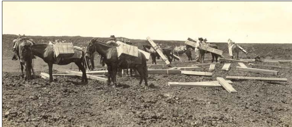
Figure 19. Unloading cabin material at summit (photo courtesy of the National Park Service, Hawaii Volcanoes National Park).
