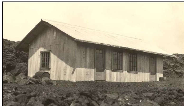
Figure 20. LCS ID 058269, Summit Rest House (ca. 1934) in its original location (photo courtesy of the National Park Service, Hawaii Volcanoes National Park).
