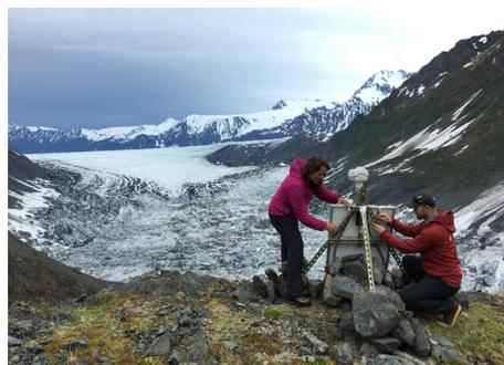
Installing the Bear Glacier ice-dammed lake camera. NPS Photo/B. Briceland.
