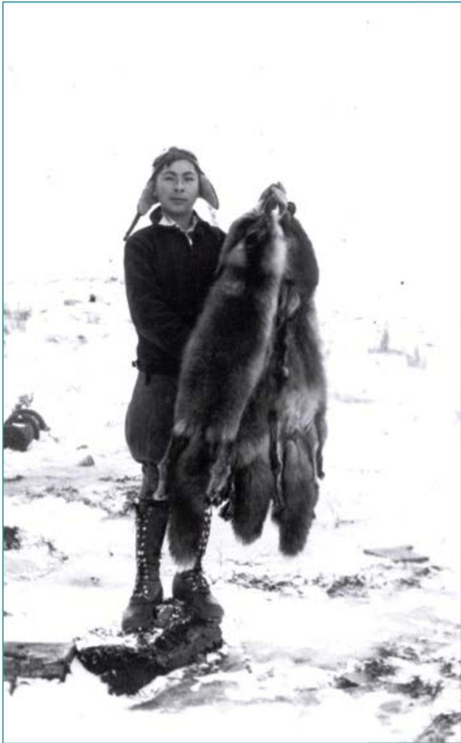
Photo 30. Charlie Roehl with fox furs at Seversen's Roadhouse. NPS photo H609.
