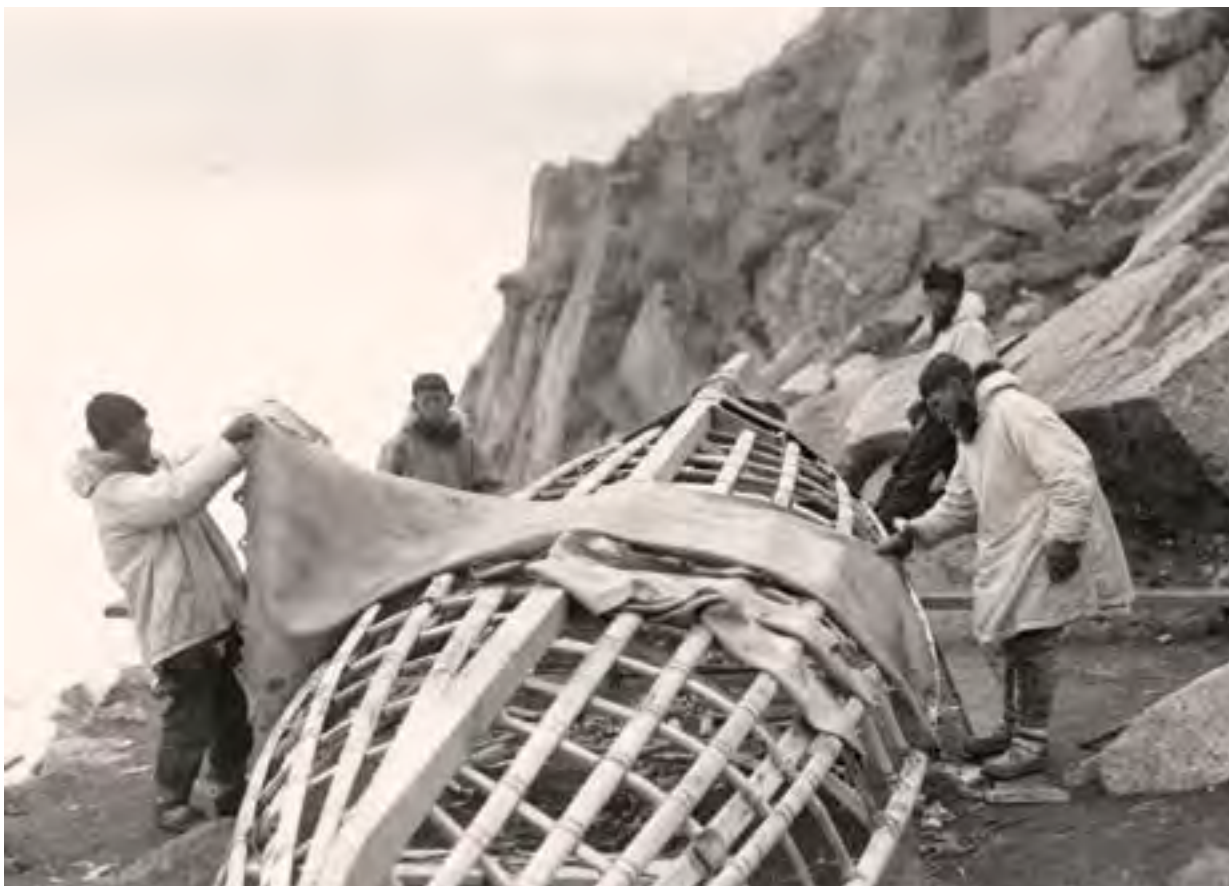
9.11 Building an umiak , using methods also employed by the Alutiiqs. The driftwood frame is complete and the men are fitting the skin cover. PHOTOGRAPH TAKEN IN 1939, LOCATION UNKNOWN. ©MARINER'S MUSEUM/CORBIS.
