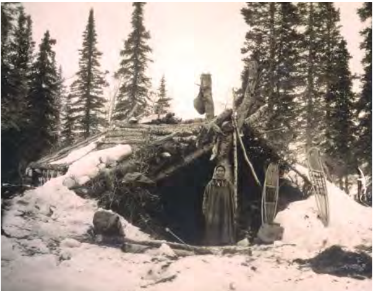
8.13 An unidentified woman stands in front of a partially constructed Dena'ina winter house on the Newhalen Portage between present-day Iliamna and the middle Newhalen River in 1908. Note the upright forked birch support and the skin-bag cache hanging from it. PHOTOGRAPH BY A. S. TULLOCH, CAPTION BY JAMES KARI. NATIONAL PARK SERVICE HISTORIC PHOTOGRAPH COLLECTION NO. H-121.
