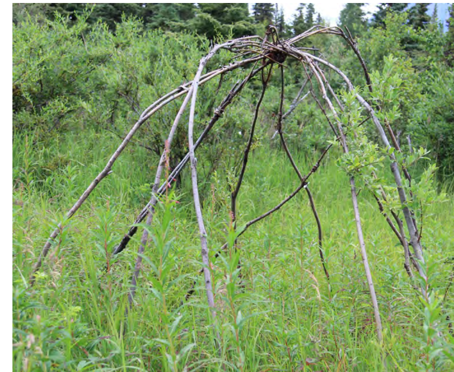
The frame of a temporary structure built of riparian willow ( Salix spp.) along the banks of Chulitna River. Cut stalks have taken root in this case, so that some supports are still living, likely becoming full shrubs over time. DOUGLAS DEUR PHOTO.
