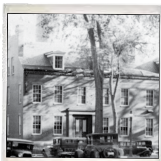
Boott Mill Agent's House
