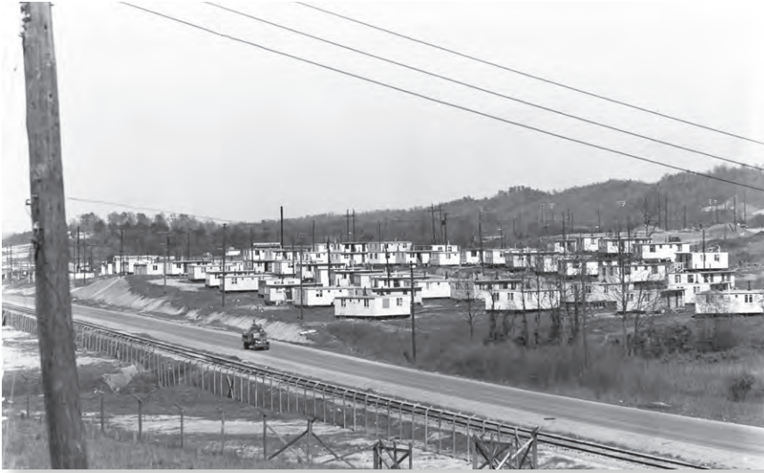
This April 1949 photo of duplex construction on Houston Ave. shows development of the newly established Scarboro community. Courtesy DOE photo collection.
