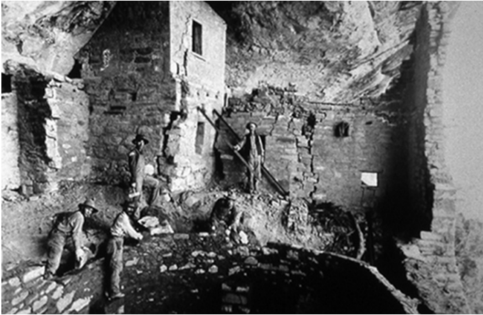
Balcony House kiva courtyard during excavation and stabilization
