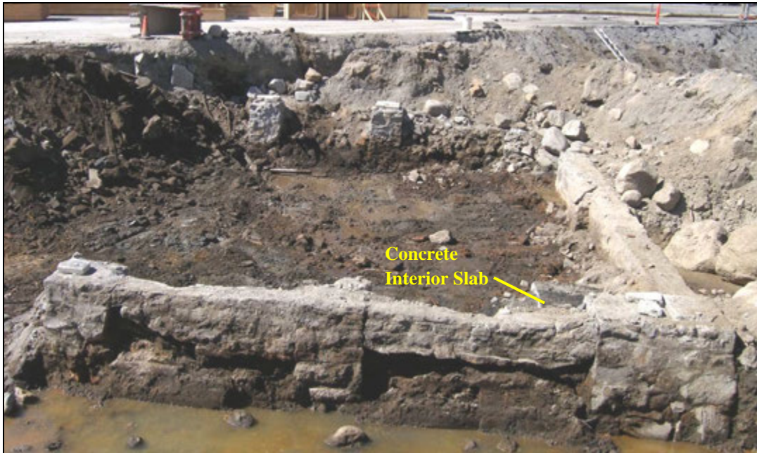
Figure 35. Paradise Camp Lodge Concrete Basement Flooring/Slab and Foundation Walls. (Photo faces SW. Slab remnant in northeast corner, oriented horizontally, and measuring approximately 3 m (L) x 2m (W) x 20cm (thick).)
