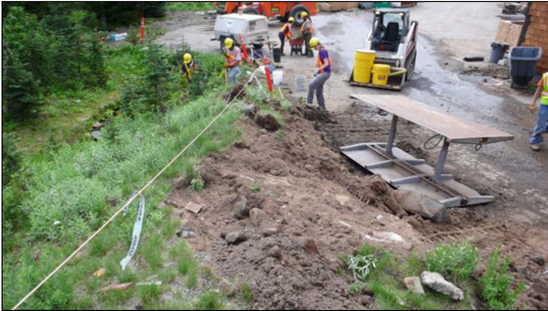
Figure 55. Tank Replacement Excavation in Vegetated Fill North of Paradise Inn
