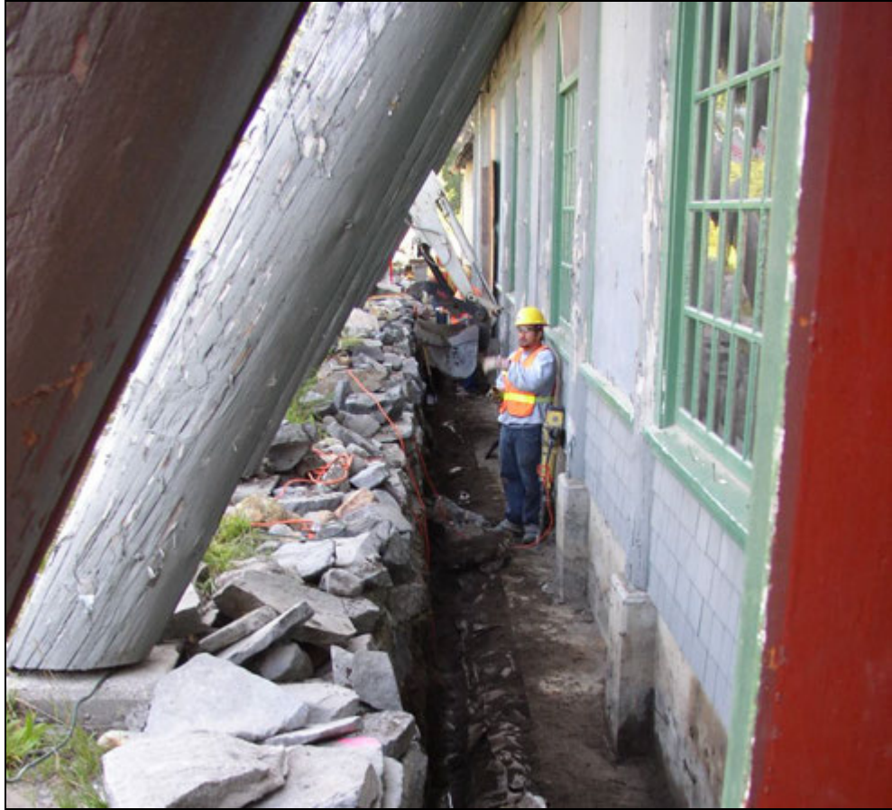
Figure 39. Paradise Inn Storm Drain Trench West of Dining Room and Kitchen
