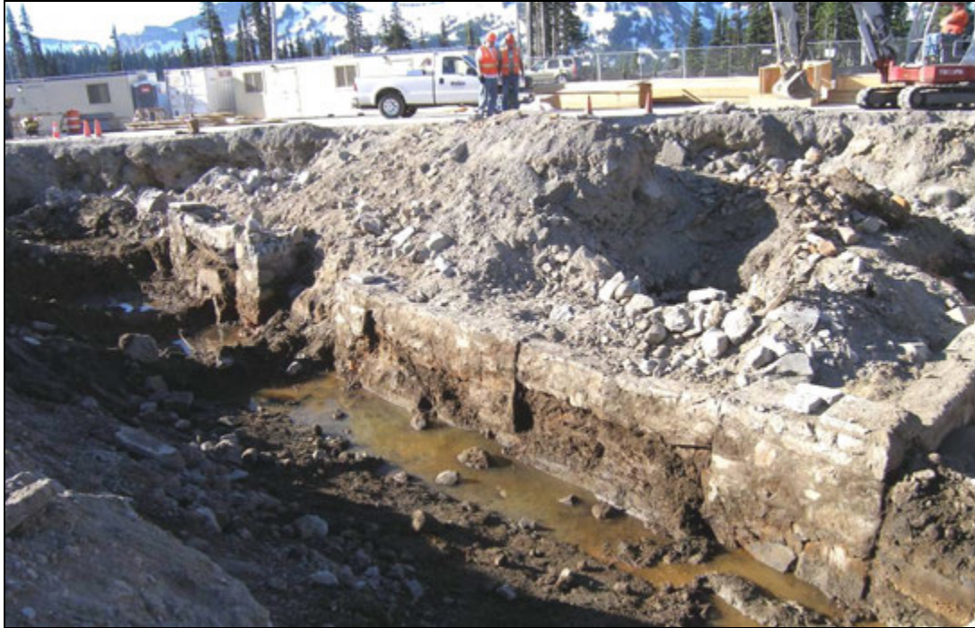
Figure 32. Paradise Camp Lodge, Exposed Eastern Foundation Wall
