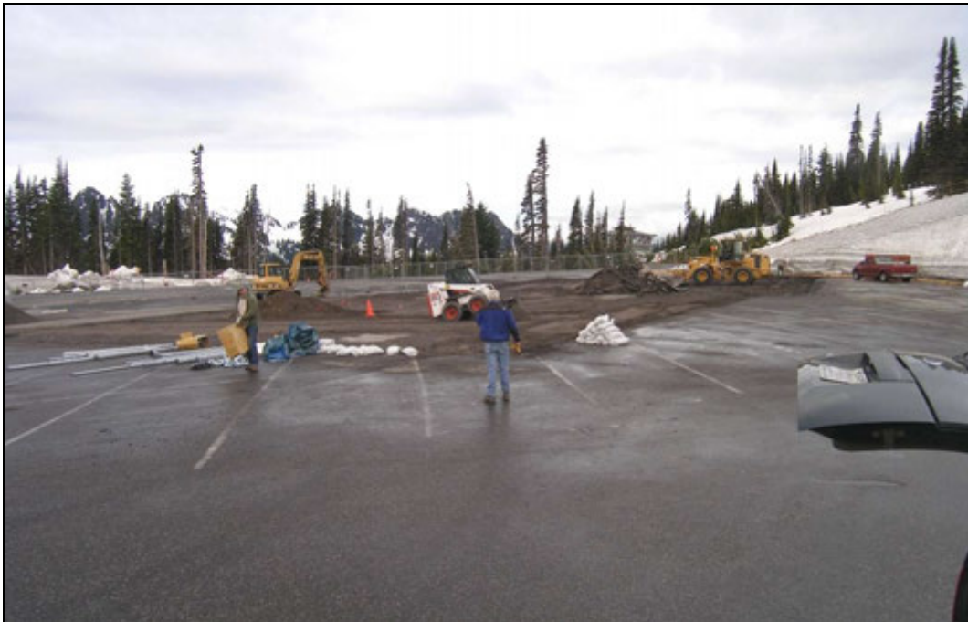
Figure 17, Asphalt Removed from the Visitor Center Footprint. (View Facing West.)
