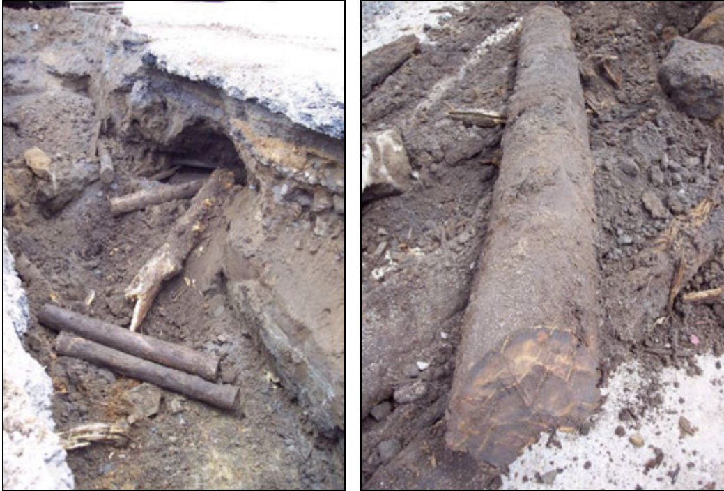
Figure 48. Log Feature 6 in Exposed Parking Area Storm Drain Trench
