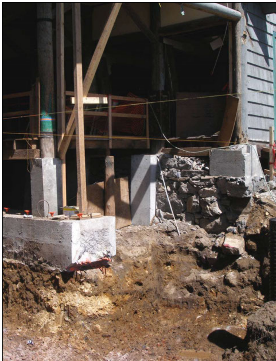
Figure 37. South Chimney Foundation Excavation
