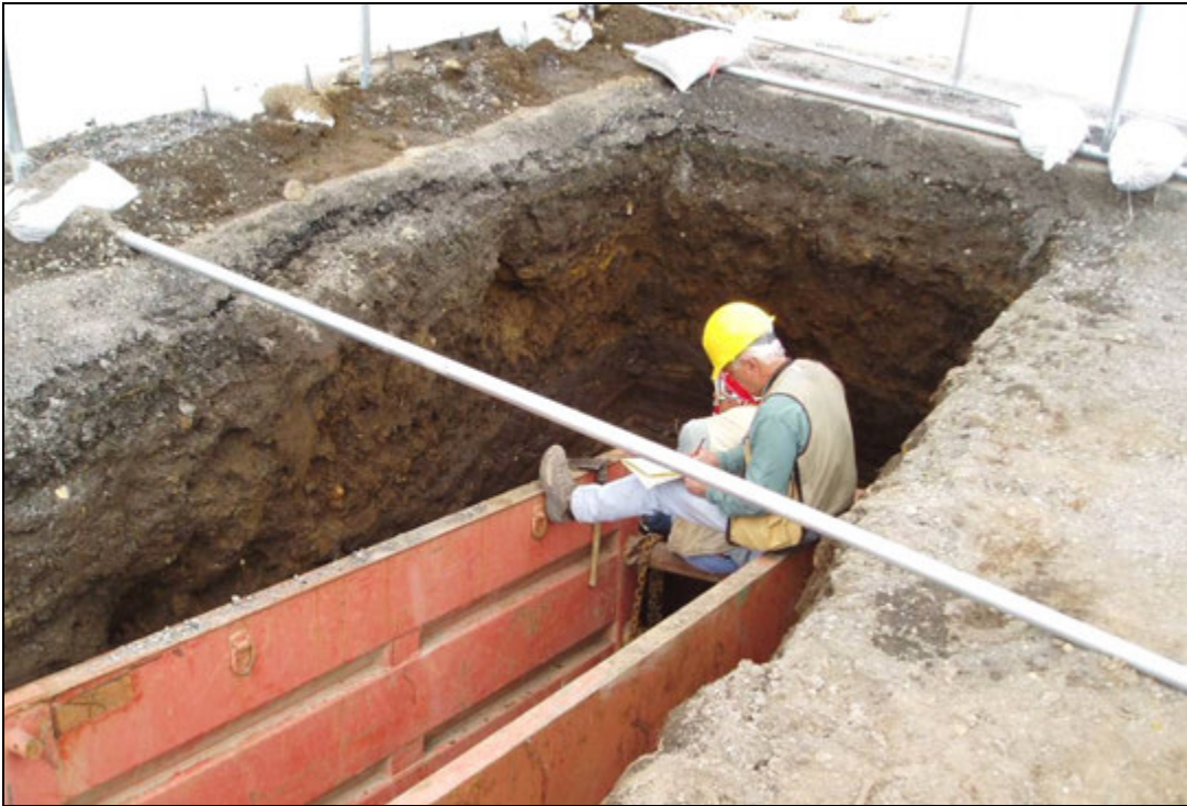
Figure 19. Upper Parking Lot Fill Layers in the Stratigraphic Trench
