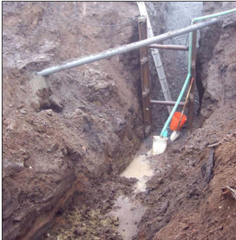
Figure 47. New Sewer Line Trenching in Progress.
