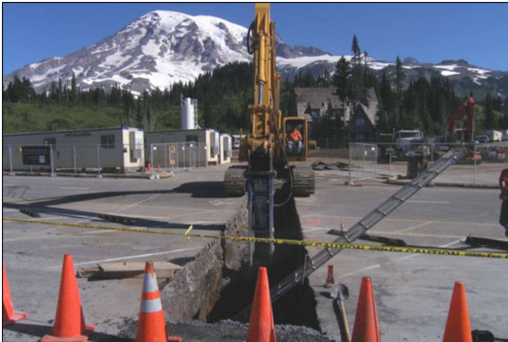
Figure 44. Trenching for Storm Drain
