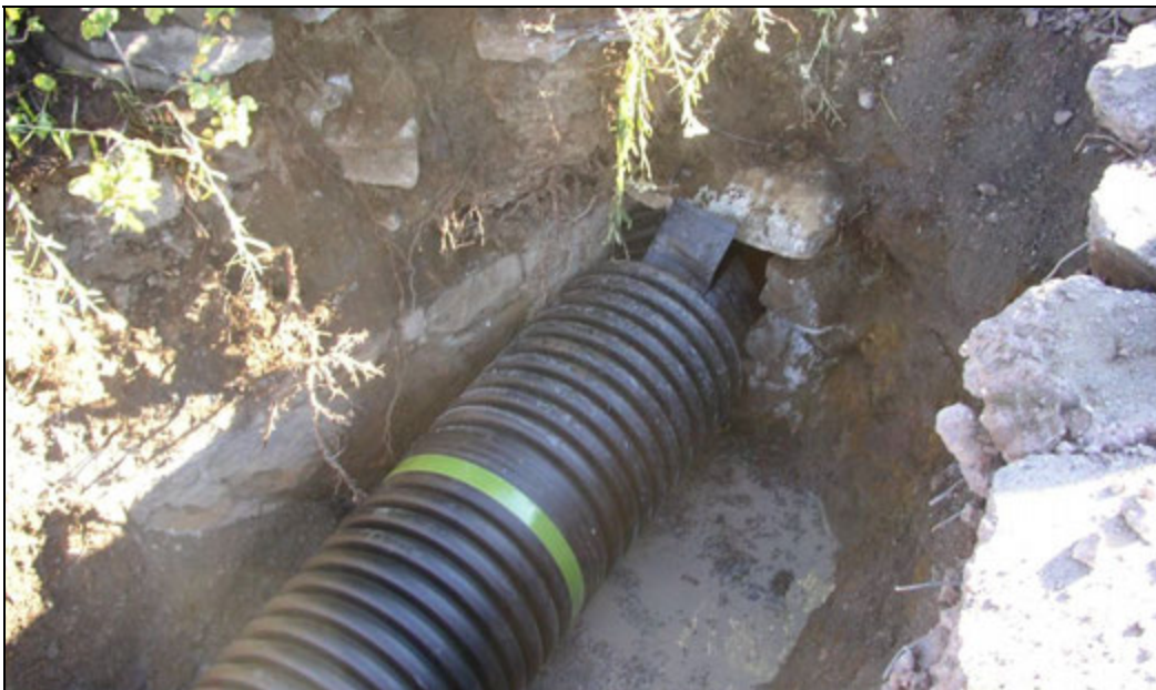
Figure 49. Slab Lined Aquaduct/Drain Feature 7.
