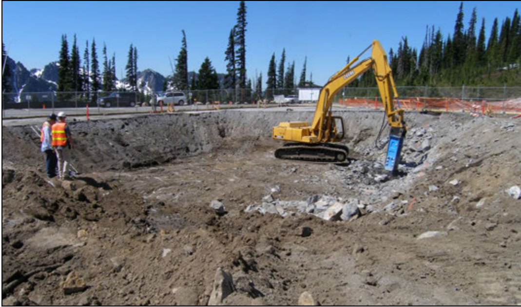
Figure 31. Excavating Paradise Visitor Center Foundation.
