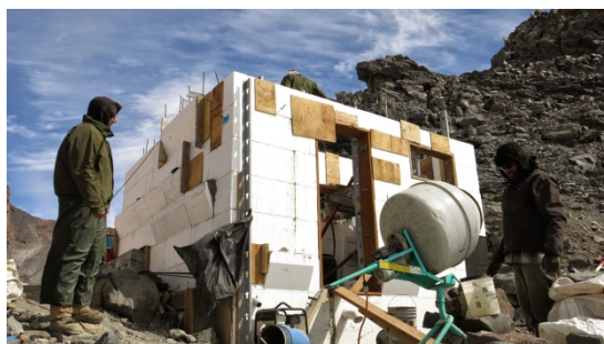
Figure 11 New toilet construction at Camp Muir
