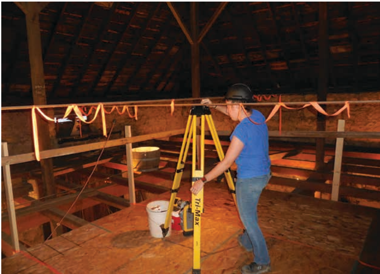
Measuring interior of the Marysville Home Station No. 1 historic barn for roof stabilization
