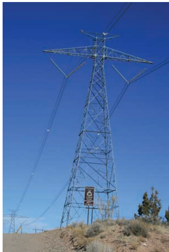
Transmission lines along the Old Spanish NHT in rural Utah
