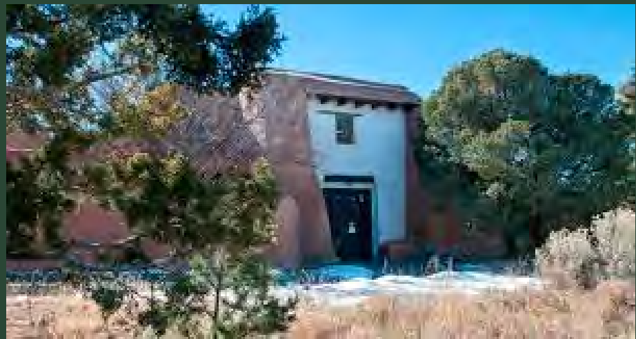
THE OLD SANTA FE TRAIL BUILDING, ON MUSEUM HILL SOUTHEAST OF DOWNTOWN SANTA FE, HAS SERVED AS THE SANTA FE OFFICES FOR TRAILS STAFF SINCE 2002. © NATIONAL PARK SERVICE
