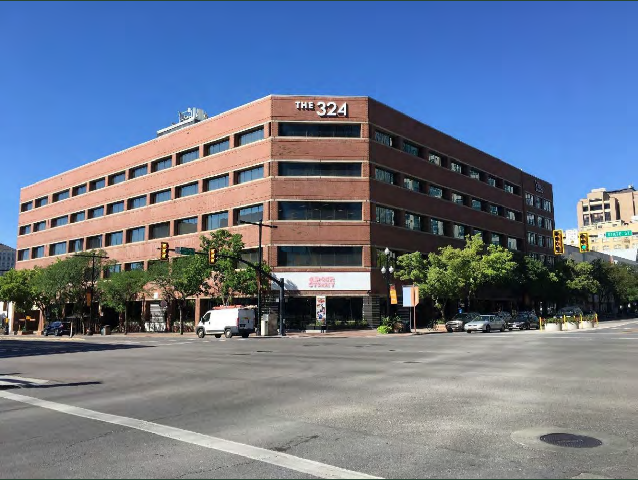
324 SOUTH STATE STREET, AT THE SOUTHWEST CORNER OF EAST BROADWAY (300 SOUTH), SERVED AS THE SALT LAKE CITY OFFICES FOR TRAILS STAFF FROM 1995 TO 2018. © NATIONAL PARK SERVICE
