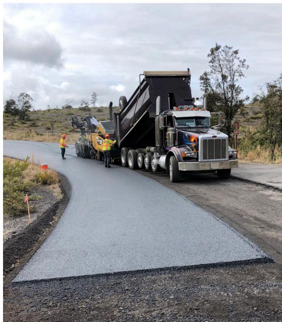
The project repaired and replaced heavily damaged pavement at multiple locations around the summit caldera. Frequently, the entire road structure was lost into deep earth cracks resulting from the volcanic collapse. Repairs included special engineering strategies such as rock scaling, installation of geotextile, and geogrid to improve resiliency of the roadways against future damage from eruptions of this volcano, one of the world's most active.
