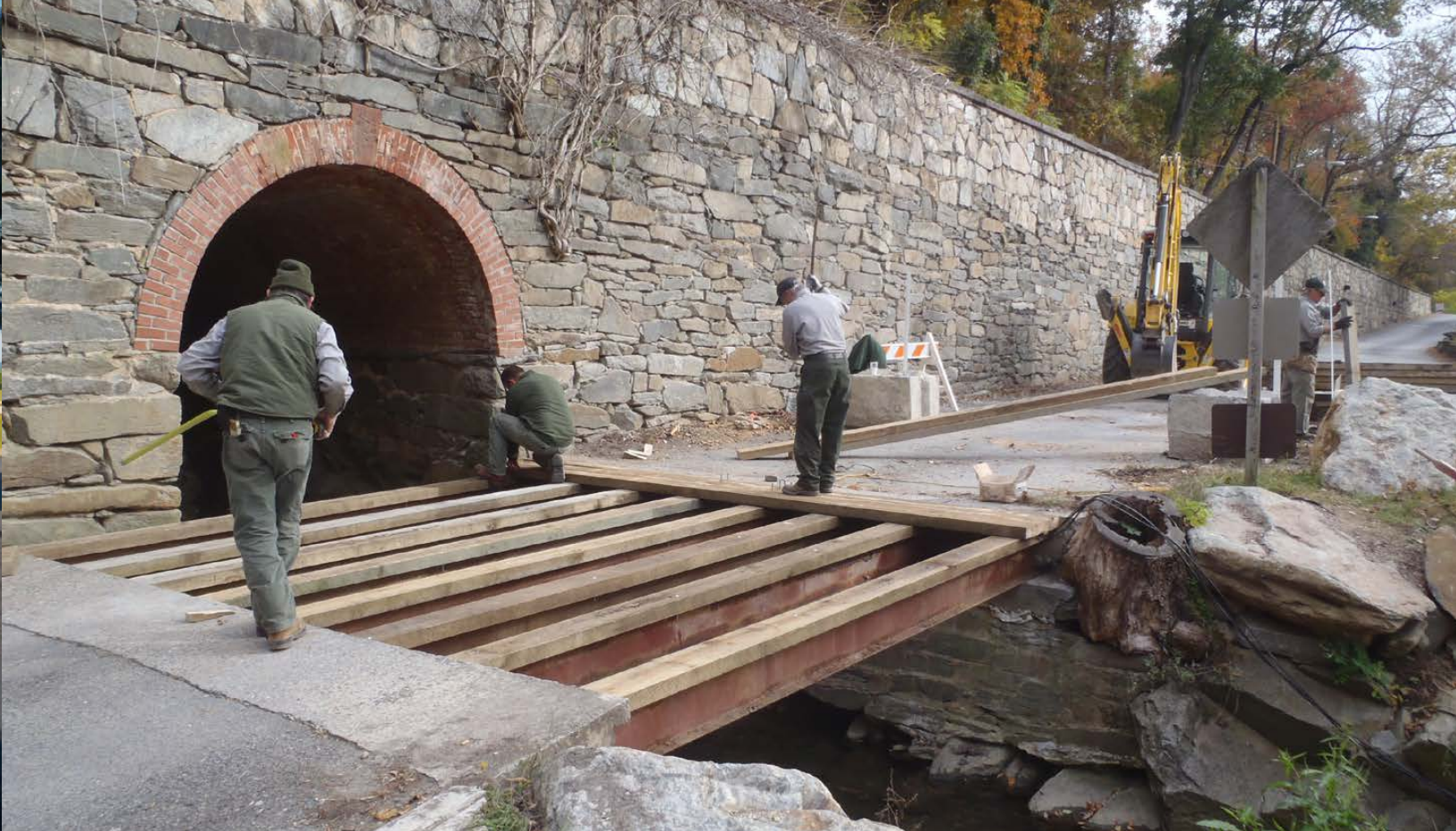
Bridge repair work in Chesapeake and Ohio Canal National Historical Park.
