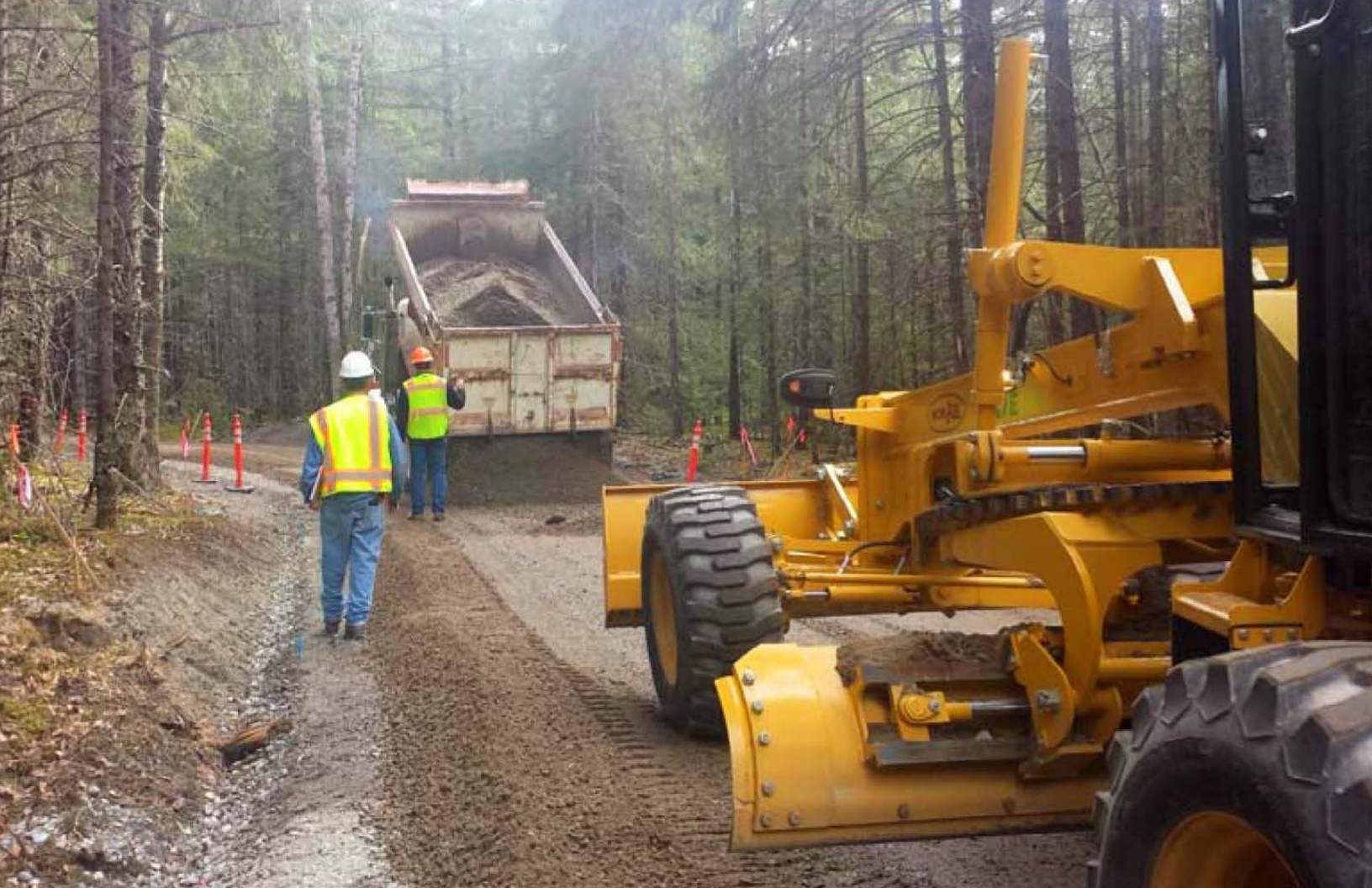
Reconstruction of Dyea Road in Klondike Gold Rush National Historical Park.
