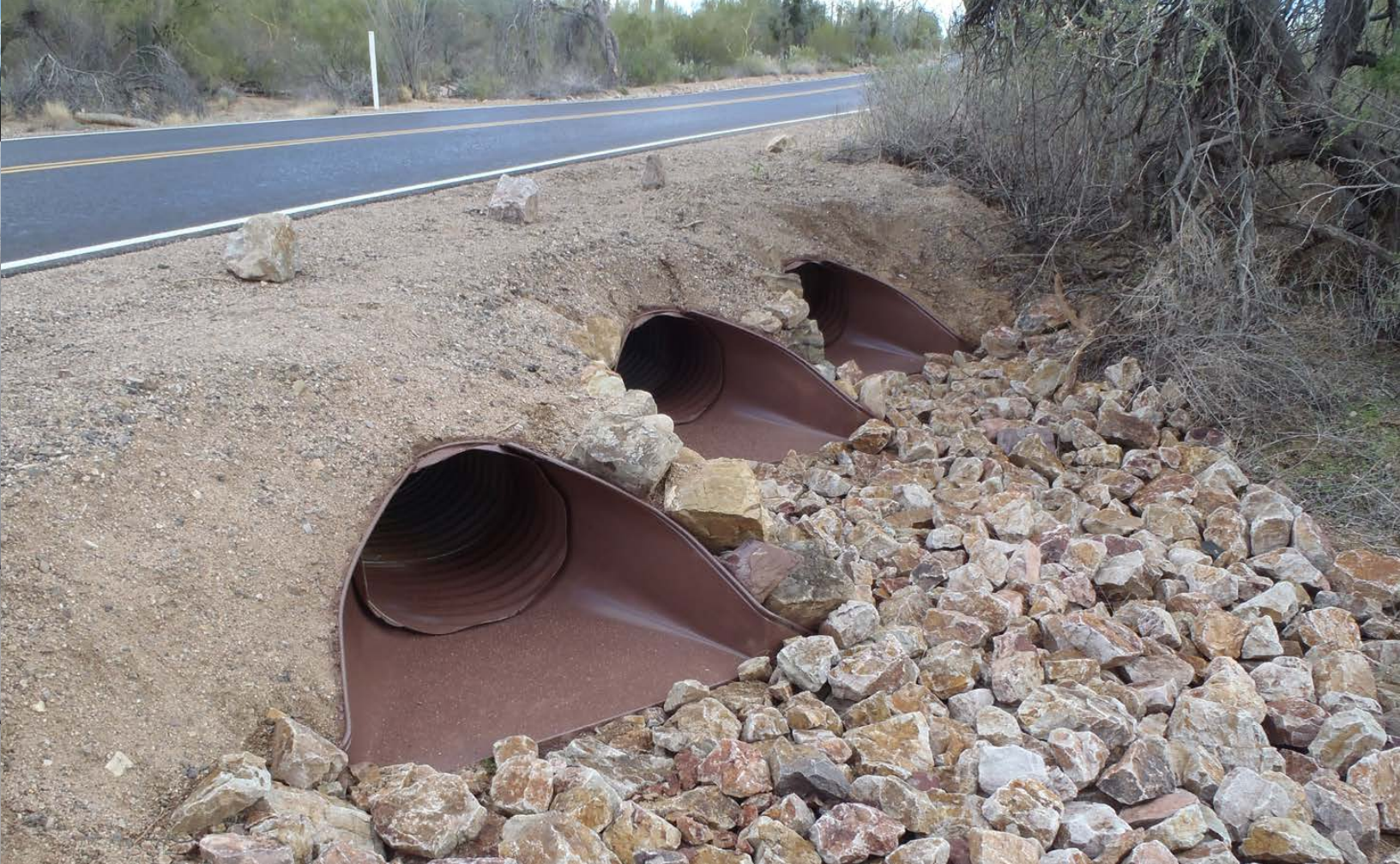
New culverts under Kinney Road in Saguaro National Park.
