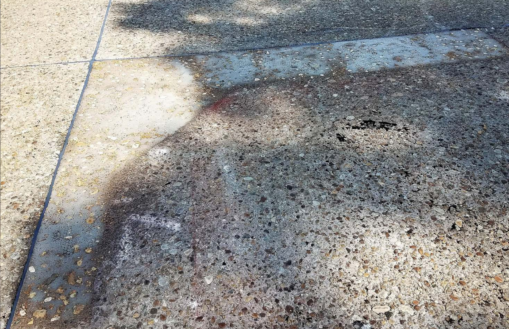
Concrete patching and joint replacement in Colonial National Historical Park.
