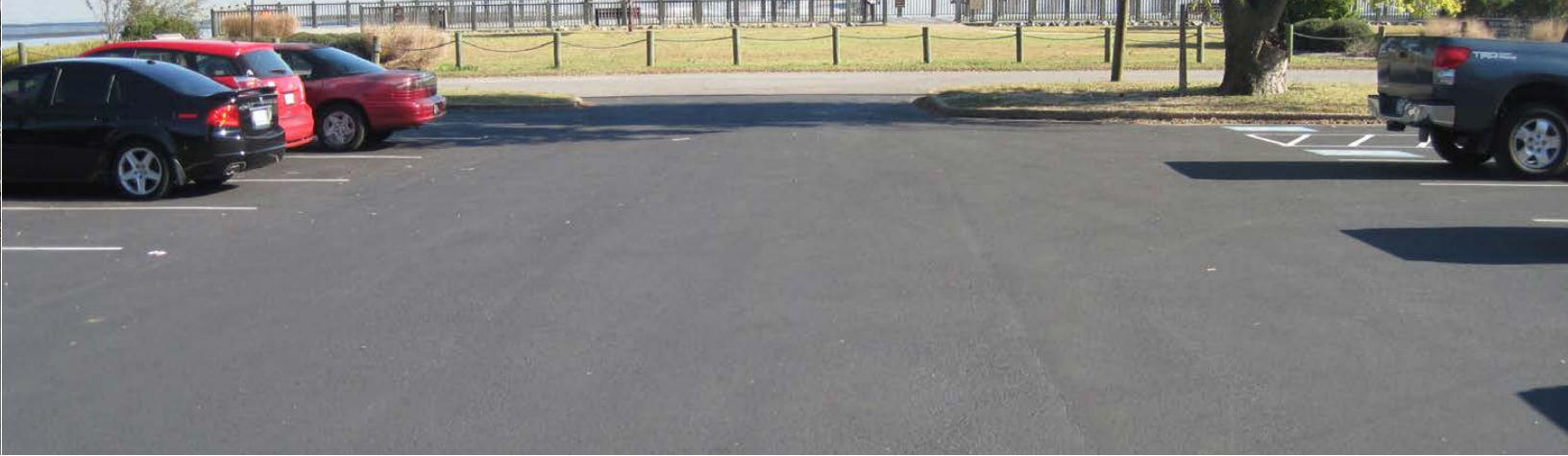
New repaved parking lot at same location at Petersburg National Battlefield and Cemetery.
