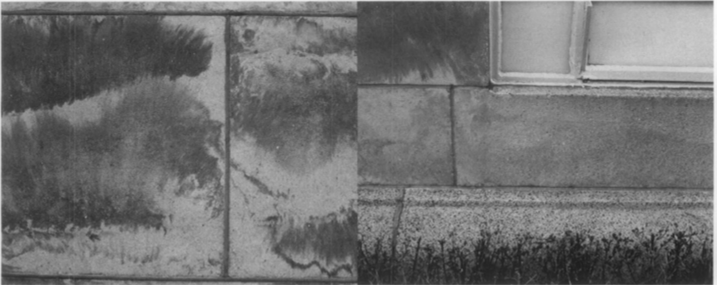
Figure 12. Elaborate pigmentation of the cementing matrix sometimes gave a rather stylized or unnatural appearance to the finished cast stone (left). Texts state that effects like this were sometimes produced by drawing strings dipped in masonry pigments across the surface of the uncured units. Cast stone, such as this, has its coloration only at the outer surface of the stone, and was not intended to be brushed or tooled to expose the aggregate. Erosion of the cementing matrix of this type of cast stone, as seen on the base of the wall (right), will result in a significant alteration of appearance.
