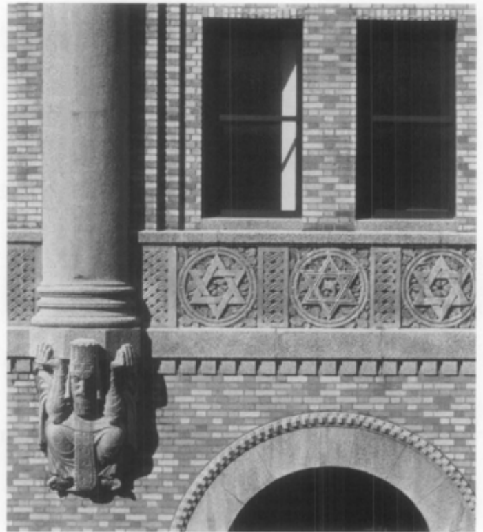
Figure 3. Sculptural ornament was frequently produced in cast stone. Repetitive detail, such as these banding course panels on the Level Club in New York City (1926), were produced much more economically than they could be in natural stone.
