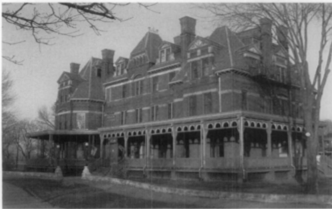
Figure 15. The historic structure report for the Hotel Florence, shown here in 1886 (upper), 1963 (center), and 2004 (lower) views, provided a basis for stabilization and repair work which has been completed. Initial phases of work addressed preservation of the building envelope, structural repairs, and limited mechanical and electrical improvements. The report also provided recommendations for future rehabilitation work that will be implemented in phases as funding becomes available. Photos: upper and center, Historic American Building Survey; lower, Wiss, Janney, Elstner Associates, Inc.
