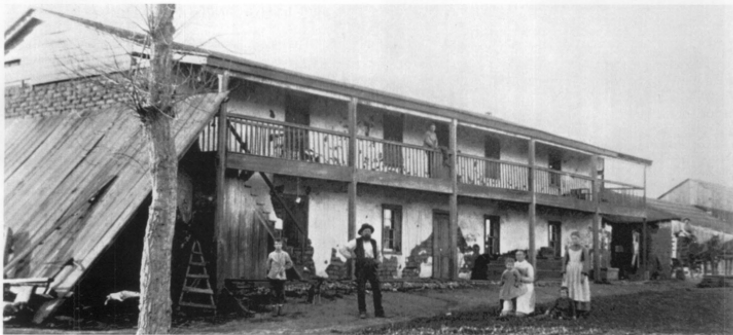
Figure 6. Historical photographs are an invaluable aid and time saver in establishing a building's original construction and evolution; in guiding the replication of missing features; and even in understanding existing material deterioration. The availability of information, such as archival photographs, surviving original architectural drawings, or HABS documentation, has a direct bearing on the cost of preparing a historic structure report. In this circa 1890 photo of the Rancho San Andrés Castro Adobe, the "lumbering up" on the south end is a character-defining feature of adobe construction, rarely seen today. Photo: Historic photograph from the Historic Structure Report for Rancho San Andrés Adobe by Edna Kimbro, State Historian, California State Parks, Monterey District.
