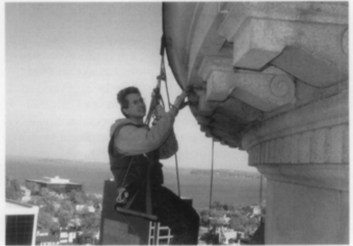
Figure 11. The use of special access methods may be necessary for close-up investigation of building elements. At the Wisconsin State Capitol, project architects and engineers used rappelling techniques. Photo: Wiss, Janney, Elstner Associates, Inc.
