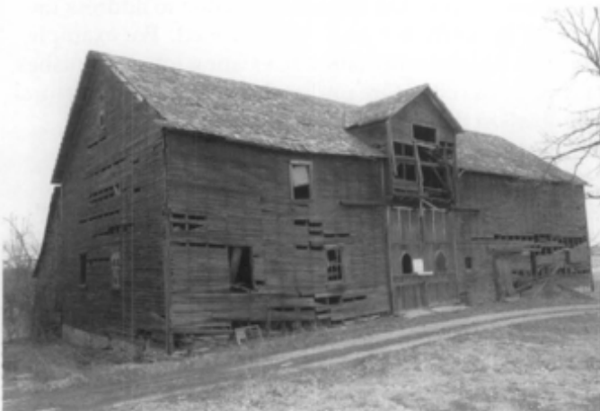
Figure 4. For small or simple projects, the project team may include only one or two specialists while complex projects may involve a large number of investigators and specialists. For example, evaluation of this barn may primarily involve a historian, an architectural conservator, and a structural engineer. Photo: Wiss, Janney, Elstner Associates, Inc.
