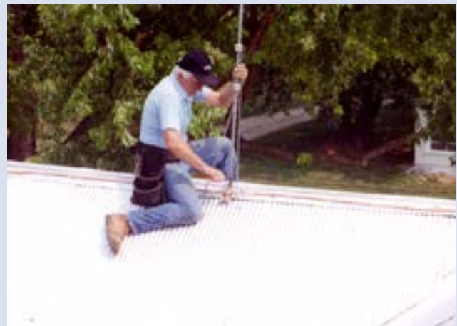
Figure B. Photo shows one of the reproduction tall lightning rods being secured in place. New cables connected the reproduction lightning rods and the modern air terminals to the down conductors that lead to the grounds. Photo: Independent Lightning Protection Company.
