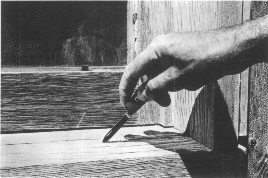
Figure 4. Close-up view of window unit treated with a paraffin-wax water-repellent *without* a chemical preservative. After 20 years' exposure, firm wood resists penetration by the knife blade. Photo: Courtesy of the Forest Products Laboratory
