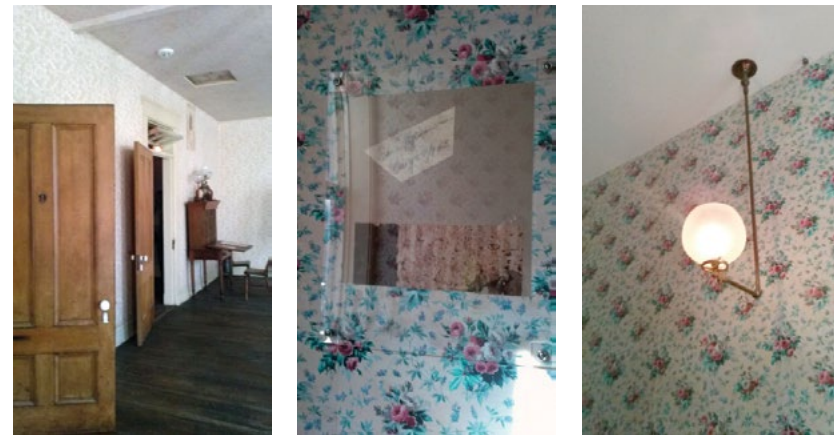
[13] (a) In the 1990s the Missing Soldier's Office—established by Clara Barton at the end of the Civil War—was discovered still extant on the third floor of a building in Washington, DC, that was slated for demolition. The office was restored to its historic appearance using physical and documentary evidence. The original numeral '9' is still on the door to the office, and wall paper was reproduced from scraps found on the walls (b-d).
