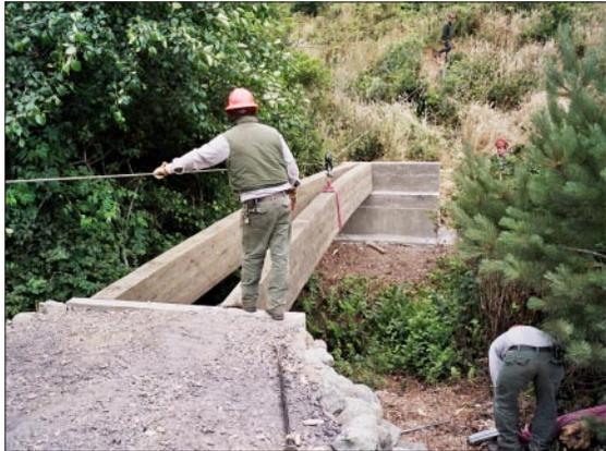
Culvert replacement with a bridge to improve passage for fish
