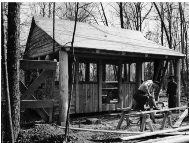
Figure 2.2 View of CCC Workers Constructing Cabins at Chopawamsic in April 1936
