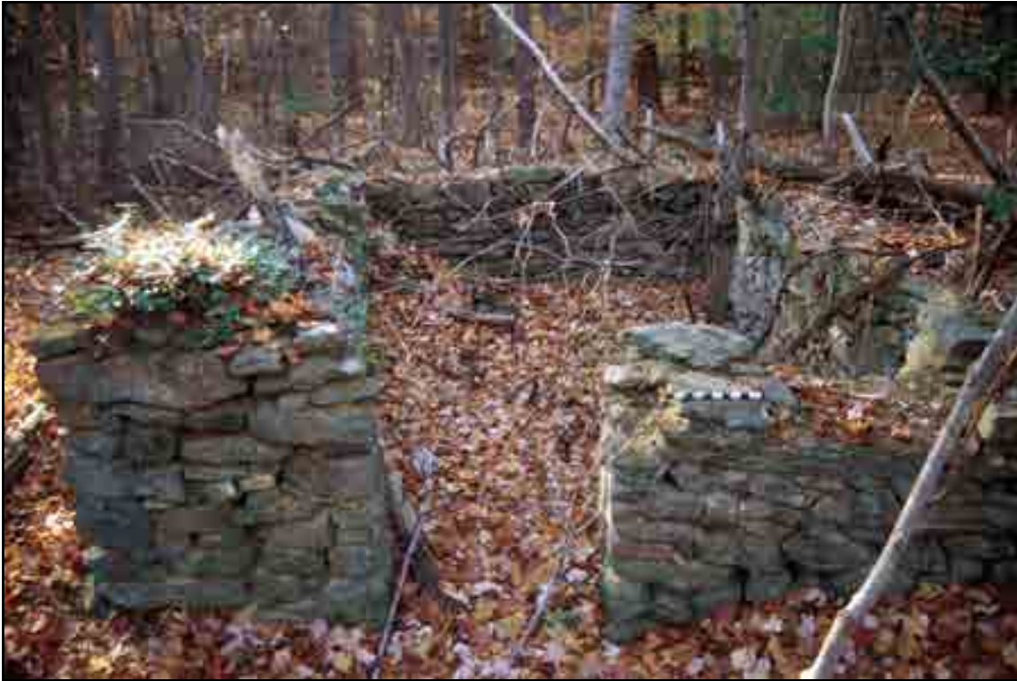
PLATE 4: Foundation of the Spring House at the Keys Site
