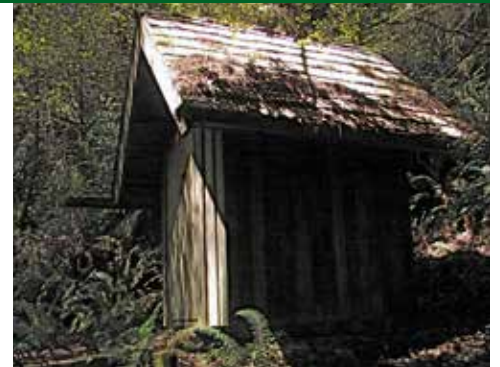
Shared pit toilet
