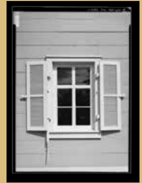
‡ Russian Bishop's House NHL window detail. Photograph Historic American Buildings Survey.
