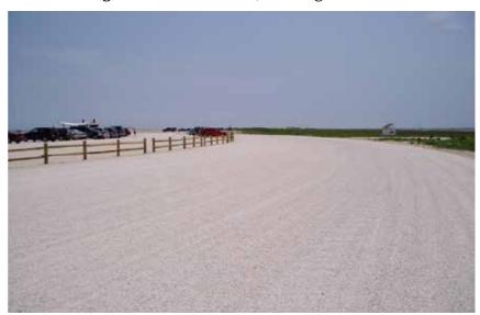
The Virginia visitor parking lot is constructed with native materials including clay and clamshell that can be reused in post-storm repairs. Image credit: Ish Ennis, NPS.
