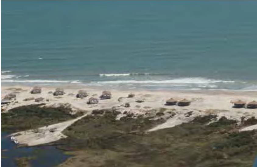
Overwash during Hurricane Irene impacted infrastructure on Long Point. Image credit: Rebecca Beavers, NPS.
