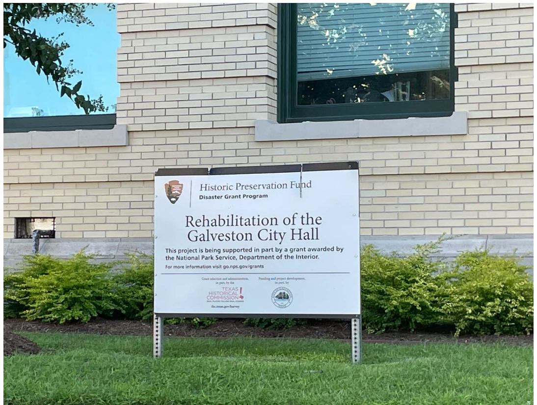
Ongoing rehabilitation of Galveston City Hall in Galveston, Texas following Hurricane Harvey in August 2017 NPS/THE TEXAS HISTORICAL COMMISSION
