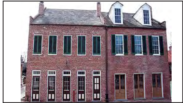
William Johnson constructed this three-story brick structure on his mother-in-law's property after an 1840 tornado destroyed much of downtown Natchez. Courtesy of National Park Service, n.d.
