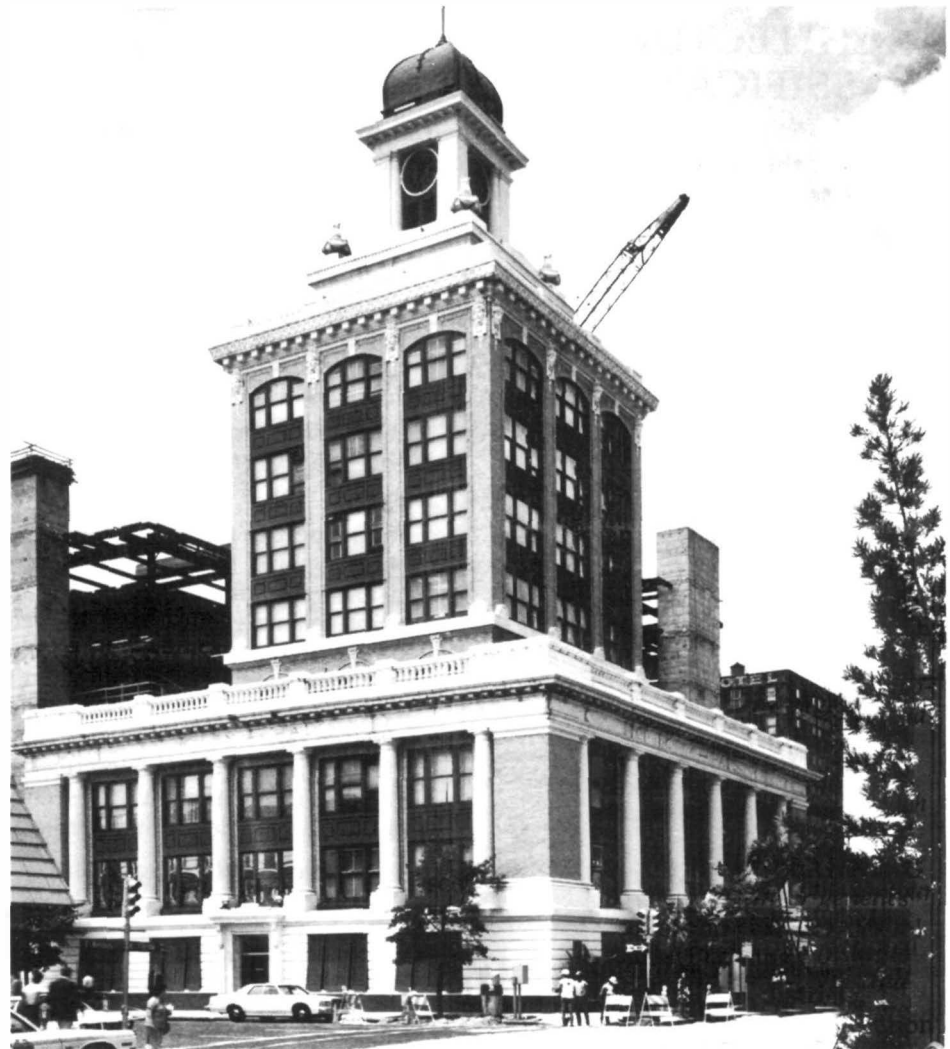
The Tampa City Hall (1914), Hillsborough County, Florida, was designed by Bonfrey and Elliott, the city's foremost architectural firm in the 20th century. It reflects the influence of both Beaux Arts Classicism and the Commercial Style. (Walter Smalling, Jr.)
