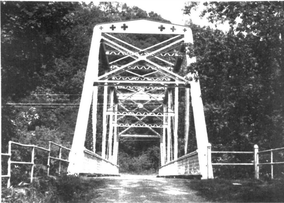
The 1898 Birmingham Bridge was nominated to the National Register of Historic Places as part of the Industrial Resources of Huntingdon County, Pennsylvania multiple property submission. Located in Birmingham, it is significant as "a fine example of one of the county's less than ten remaining pin-connected Pratt through truss bridges built in the late 1800s." (Nancy Shedd )
