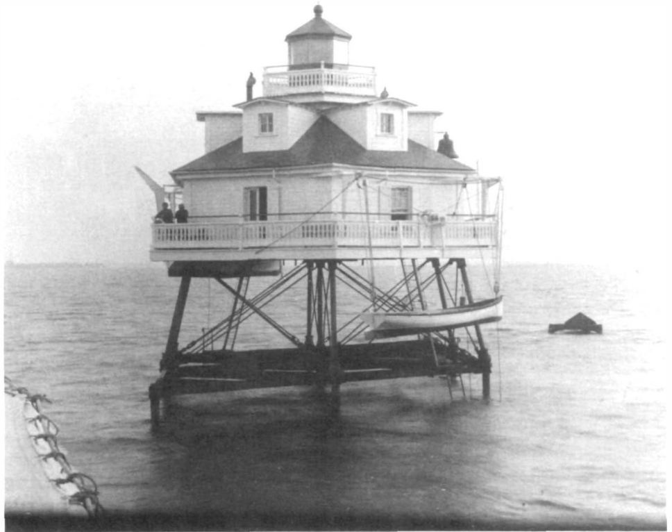
Thomas Point Shoals Light Station, standing in Maryland's Chesapeake Bay, is a hexagonal screwpile, offshore light. Screwpile refers to the nine metal pilings, tipped with two blades arranged in screw fashion, which support the structure. This method of anchoring an aid to navigation was most appropriate for the sandy, muddy bottom of the bay. In this historic photograph, taken in 1885, ten years after the completion of the light, its roof is topped with dormers and a steel octagonal cupola containing the light. (U.S. Coast Guard)
