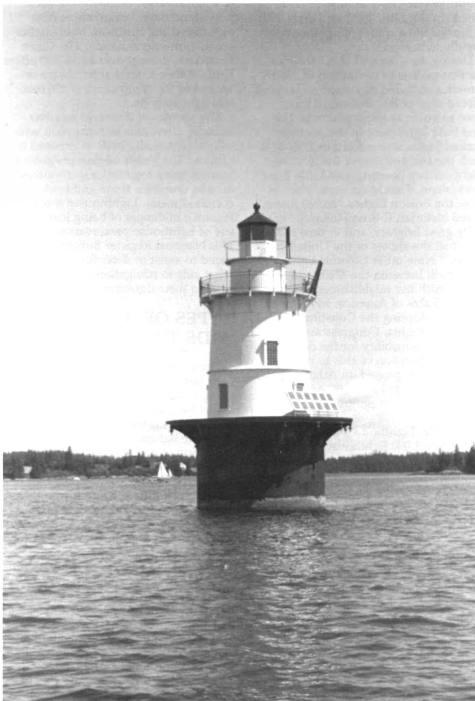
The Goose Rocks Light Station marks the east entrance to the Fox Island thoroughfare between Vinalhaven and North Haven Islands in Maine. The caisson or sparkplug light, constructed in 1890, stands on a shallow rock ledge. Within its walls are the keeper's quarters and the storage facility. The light guides not only cargo ships but pleasure vessels as well. The two islands attracted many summer tourists with numerous hotels and cottages built to serve the growing resort communities. (Roger G. Reed)
