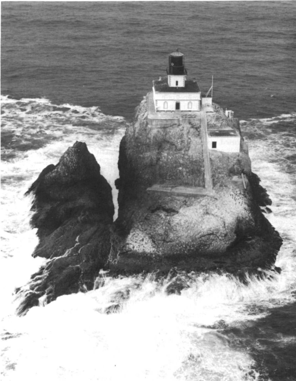
Tillamook Rock Lighthouse is significant as Oregon's only offshore light and the fourth oldest of nine lighthouses now standing on the State's coast line. Its construction, completed in 1881, was an engineering feat involving hazardous landings of workers and materials by derrick and breeches buoy from a lighthouse tender anchored off the rock. Its isolated and exposed position atop a solid basalt islet more than a mile offshore made it not only an extremely lonely post for its tenders but also one of the most challenging. The powerful beam has guided thousands of ships safely past one of the most hazardous sections of coast line on the continental United States and into the Columbia River shipping lanes, integral to the economic history of Oregon and the Northwest. (Seaside Photo)
