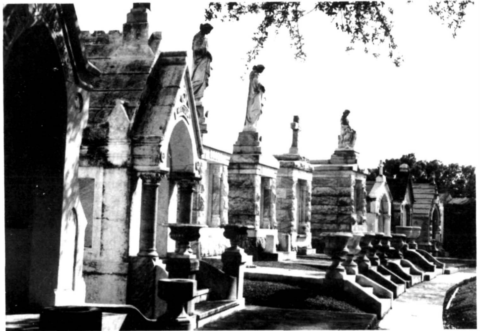
Cultural and environmental factors can be important in understanding cemeteries. In southern Louisiana, cemeteries such as the Metairie Cemetery in New Orleans, Orleans Parish, reflect high-style French funerary architecture. At the same time, the tradition of building burial vaults above ground was well-suited to the high water table of the delta region. (Donna Fricker, 1991)
