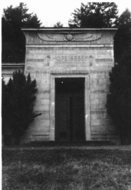
A principal contributing feature of the Masonic Cemetery in Eugene, Lane County, Oregon, is the Hope Abbey Mausoleum, which meets Criterion C as the State's only truly monumental example of the Egyptian style. (Richard Roblyer, 1980)
