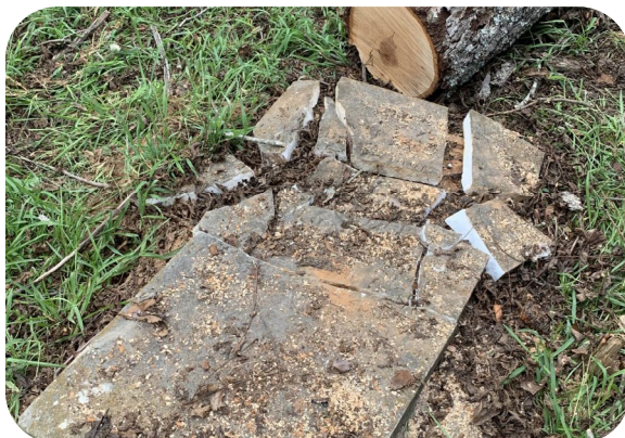
(From top to bottom) A large tree is toppled in the middle of a cemetery. Temporary shoring is used to stabilize a damaged mausoleum after a storm. A stone is damaged from a toppled tree.
