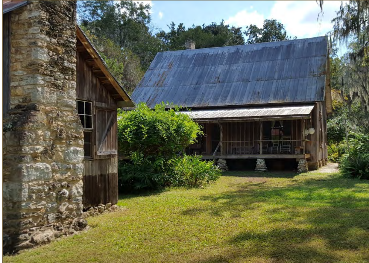
Rear elevation of main house (background) and kitchen/dining room (foreground)
