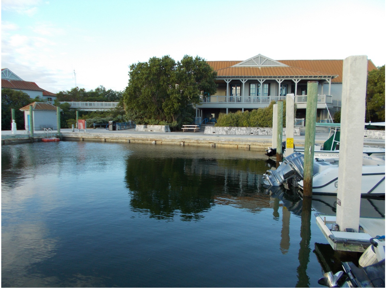
Figure 24. View (to the west) of the main bulkhead of the visitor center harbor. The bulkhead sits upon what was once the sandy beach at Homestead Bayfront Beach North.
