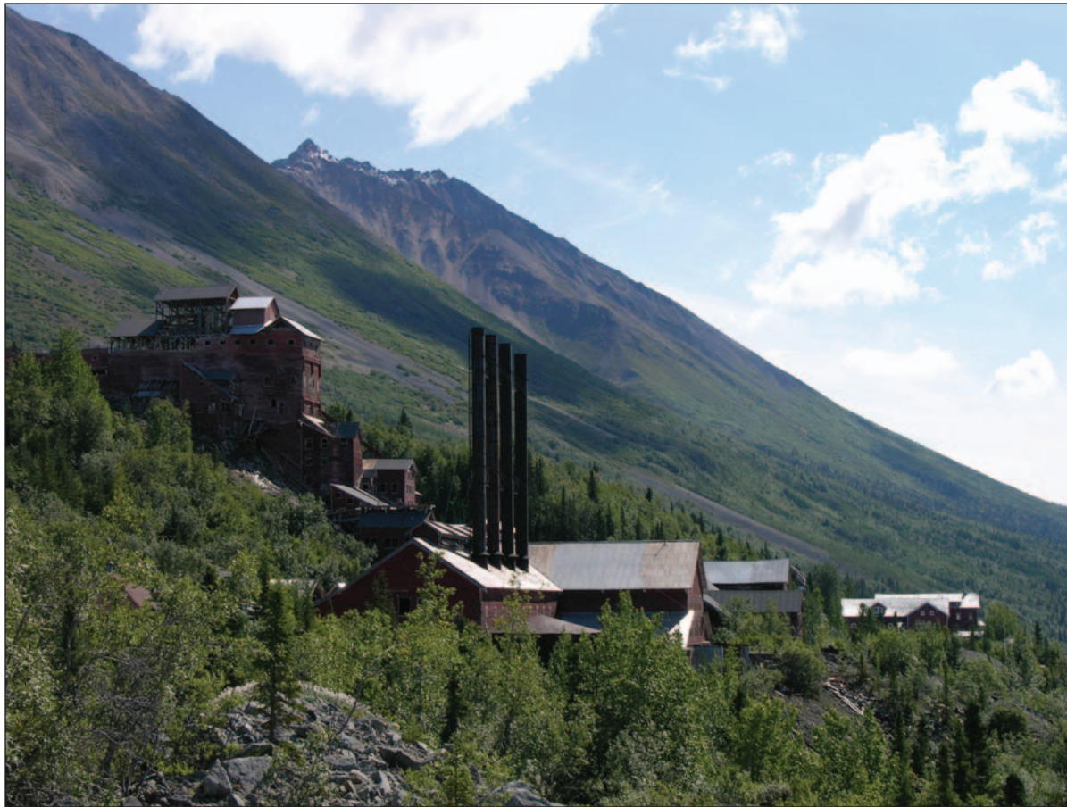
View of Mill from overlook - NPS photo Carol Harding
