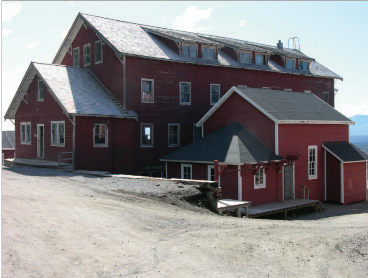
West Bunkhouse & Refrigeration Plant - NPS photo Carol Harding
