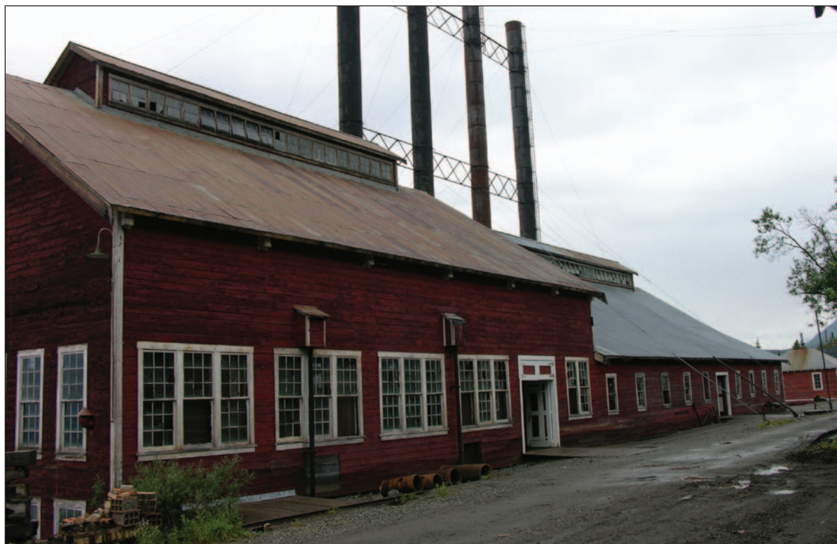
Power Plant - NPS Carol Harding
