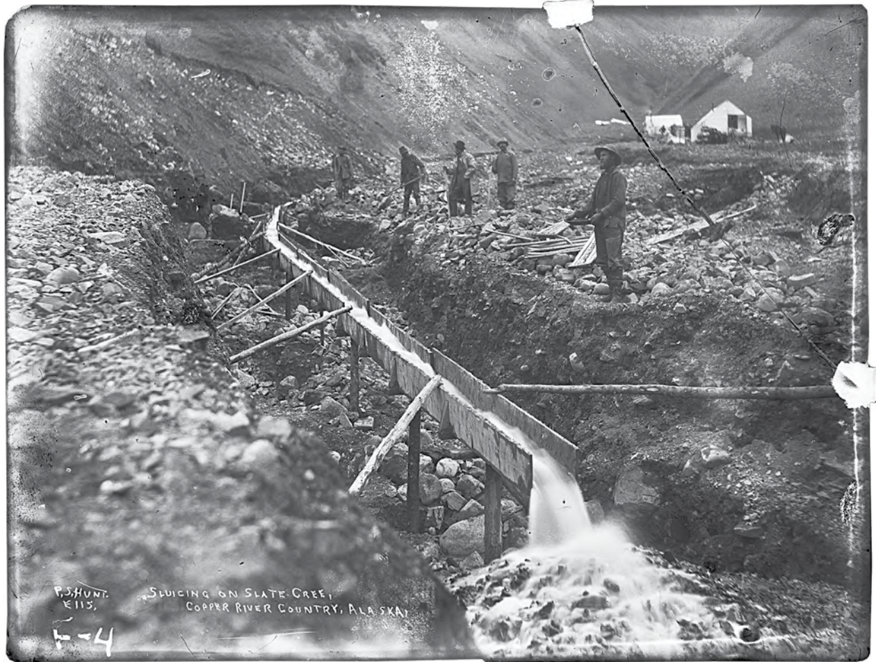
Figure 49: View of miners using sluice to mine for gold, Slate Creek, Chistochina District, Alaska. Cary-Henderson Collection, Anchorage Museum, B1962.001A.115.
