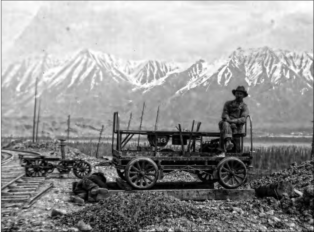
Fred Ahrens, McCarthy Section Foreman for the CR&NW Railroad, circa 1920. Courtesy of Dick Anderson.
