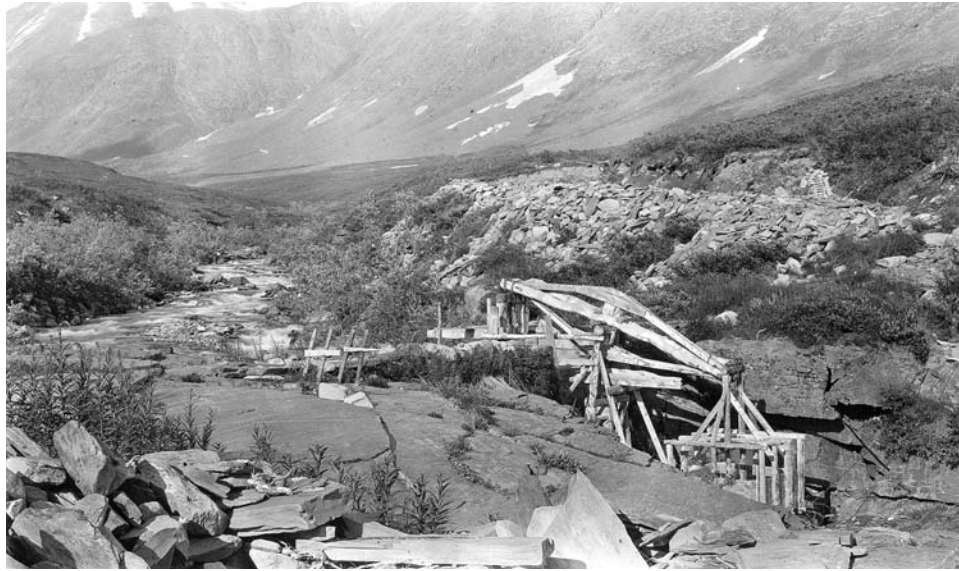
Figure 12: Early placer miners used self-emptying "boomer" dams, like this one in the Bremner district, to remove overburden. Fred Moffit Collection, U.S. Geological Survey Photo Library, Denver
