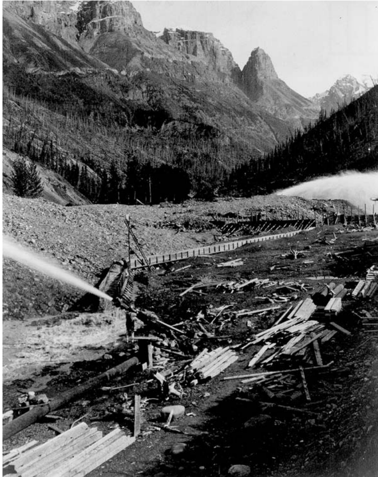
Figure 10: Placer miners, like these on Dan Creek in 1916, often used pressurized water to move overburden off the bedrock. Special Collections Division, University of Washington Libraries, Seattle
