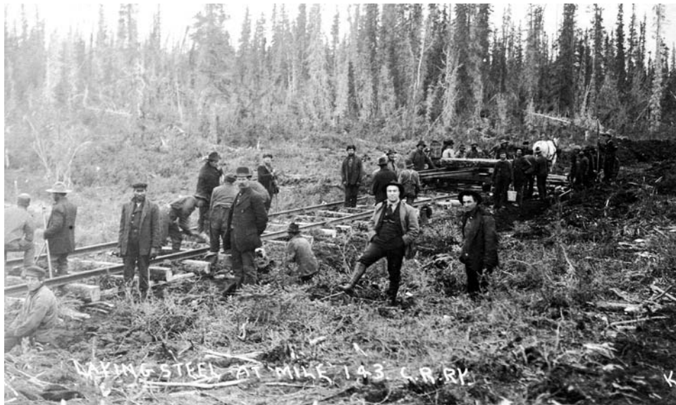
Figure 5: Laying track east of Chitina in 1910 Photo from author's collection
