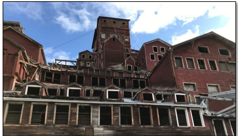
Picture of the Kennecott Mill Building
