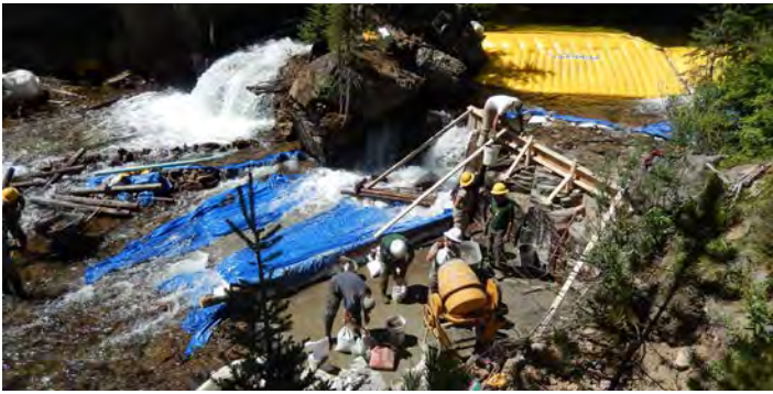
Intermountain Restoration modified an existing waterfall to form a barrier during 2013.
