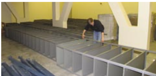
Shelving had to be purchased, assembled, installed, and cleaned before anything could go on it.
