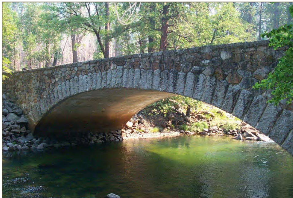
Photo F-1. Pohono Bridge: Contributing Structure in the Yosemite Valley Historic District and Yosemite Valley Bridges.
