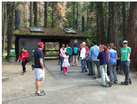
EXISTING COMFORT STATION AT BRIDALVEIL FALL
