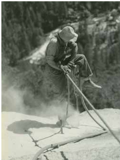
Construction of the Big Oak Flat Road, June 9, 1936. Negative RL-8702.
