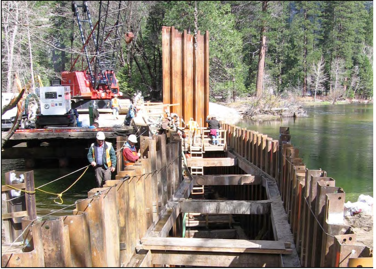
River Crossing to Consolidate Utility Lines
