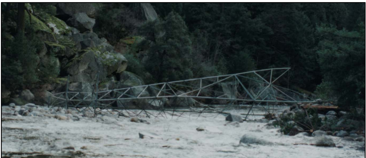
Downed Electrical Tower in Merced River
