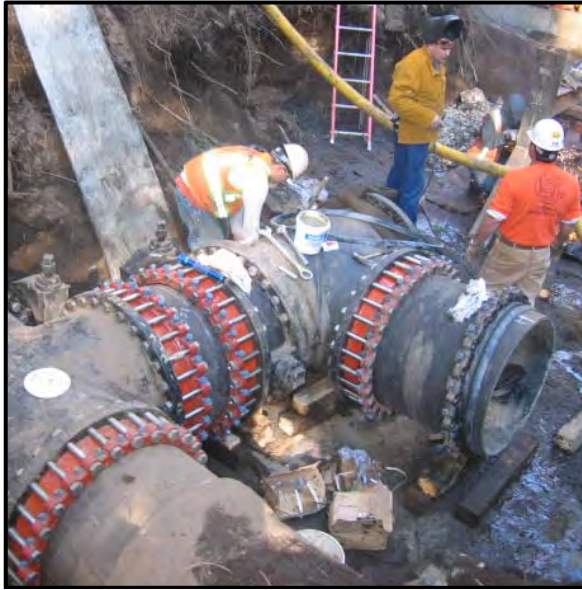
Installation of New Water Main
