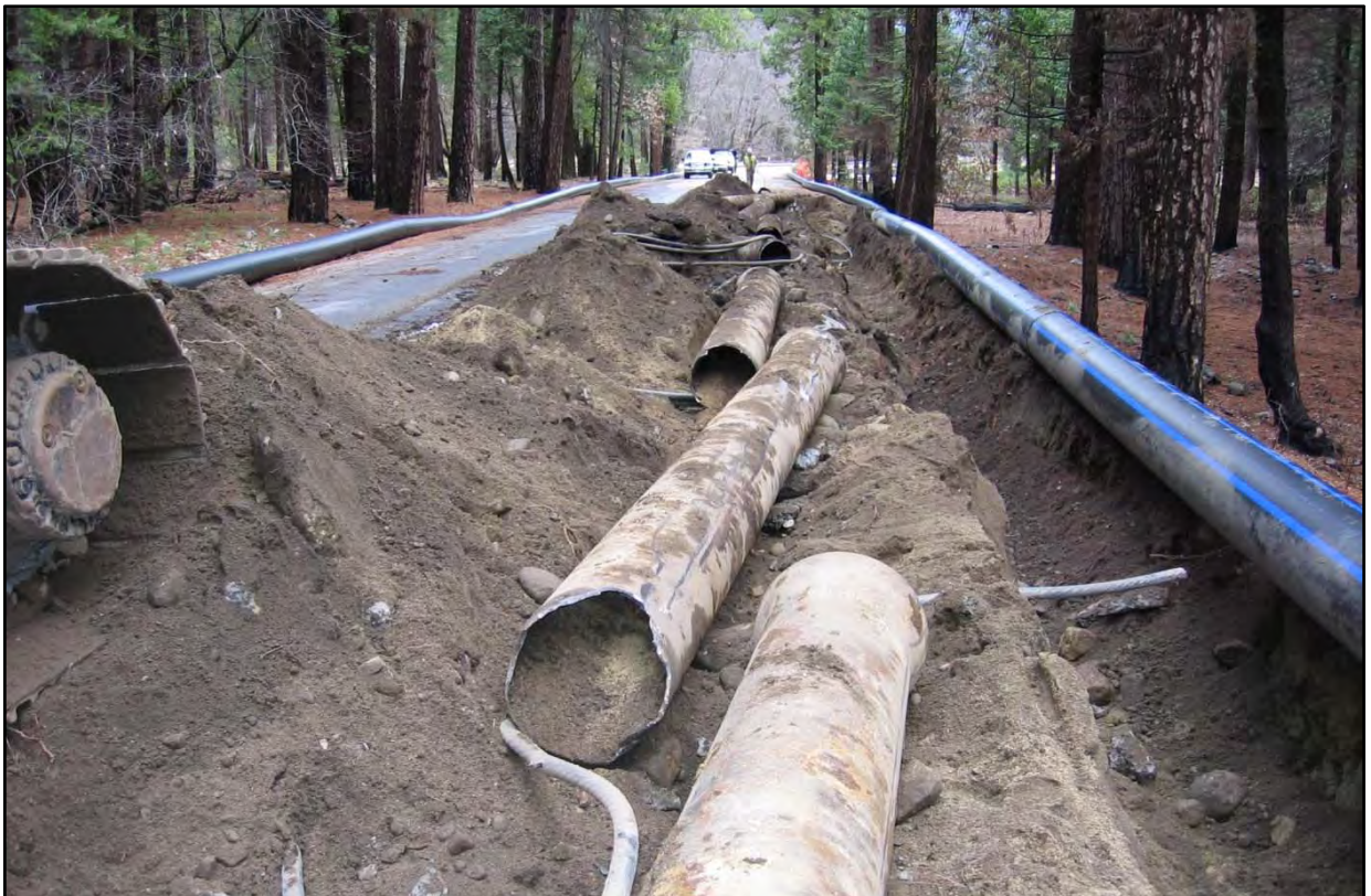
Post-Flood Sewer Line Replacement
