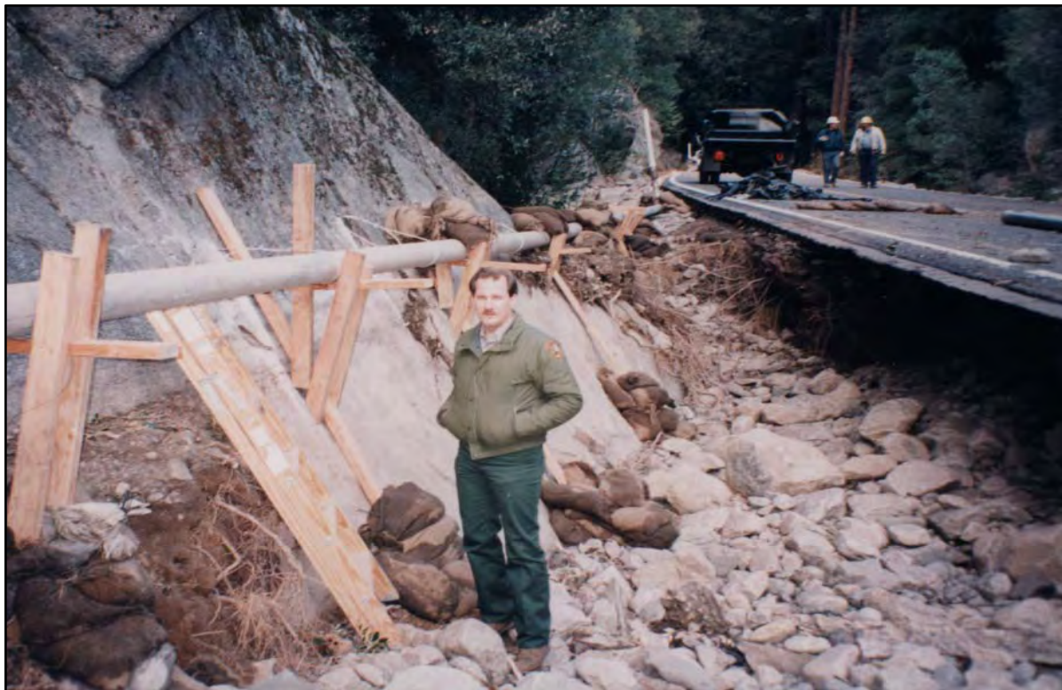
Temporary Sewer Line at Cascades
