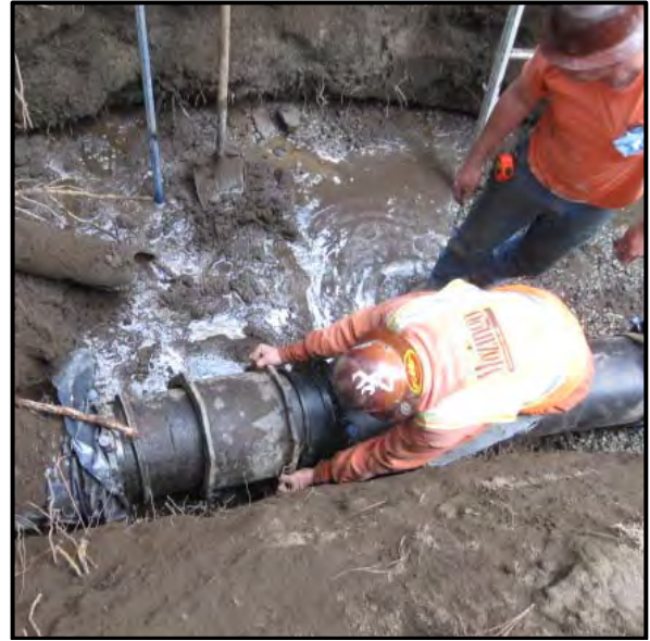
Installation of New Sewer Main
