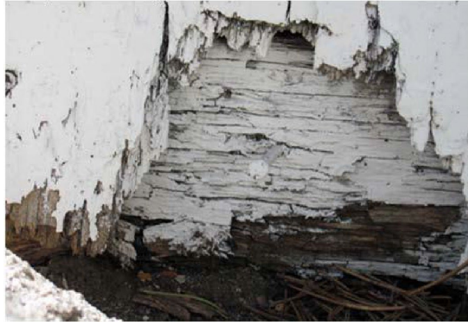
Figure 8. Decayed exterior wall
