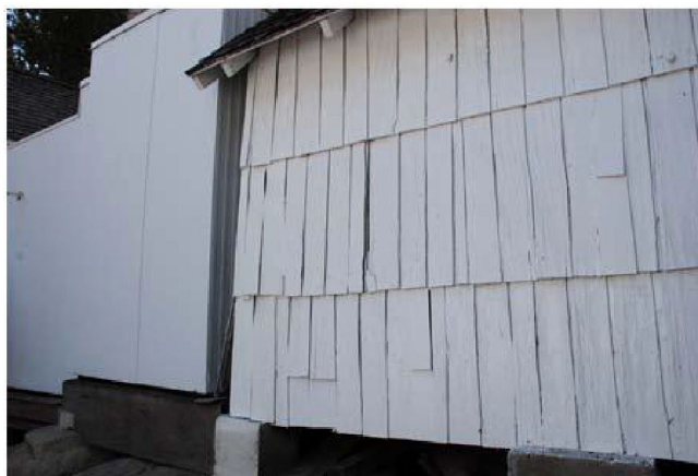
Figure 7. Deteriorating wood-shingle siding
