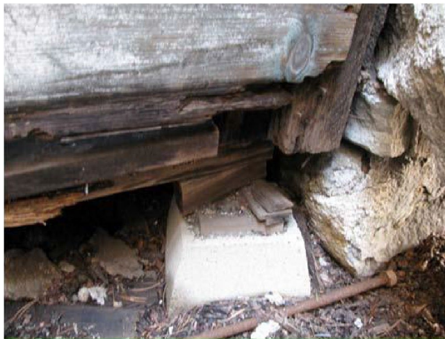
Figure 6. Erosion and settling of foundations
