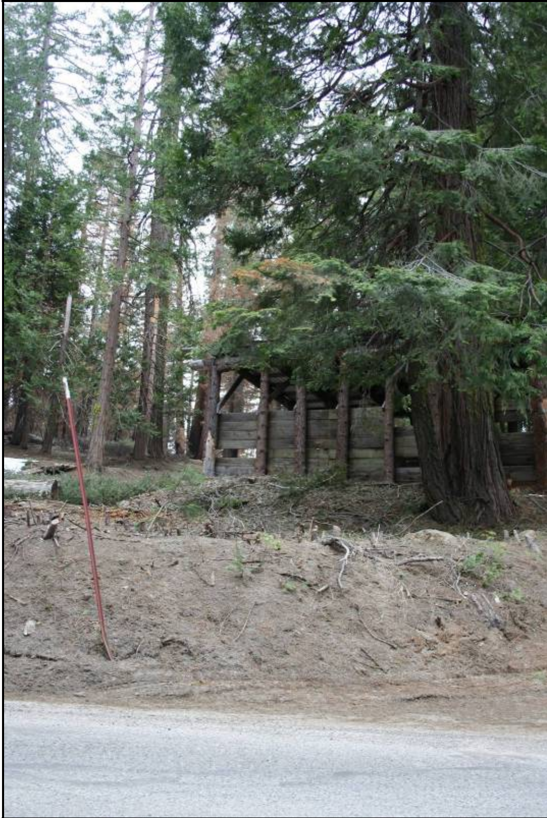
Photo HR-2: View of Modern Sand Shed from Henness Ridge Road (Viewpoint B)
