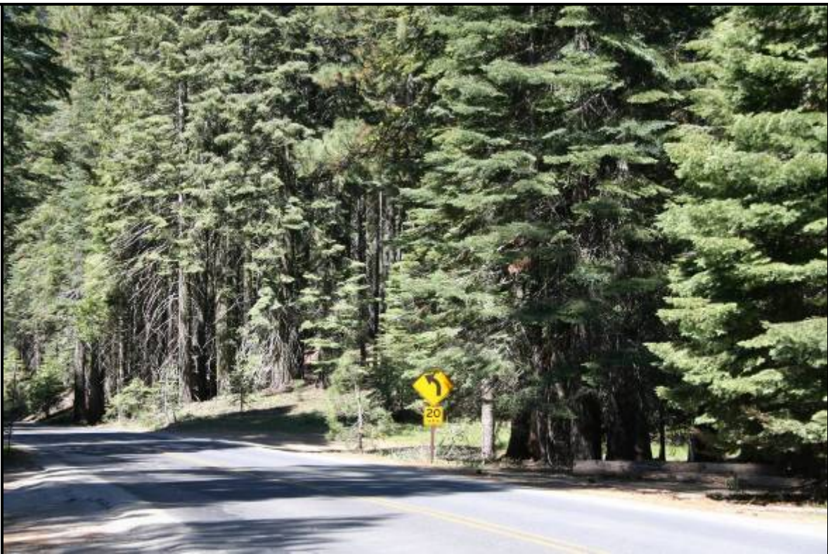
Photo CF-3: View to South of Tioga Road Adjacent to Crane Flat from Viewpoint C
