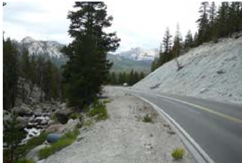
Fine soils along a portion of Tioga Road can contribute to river turbidity during storm events.
