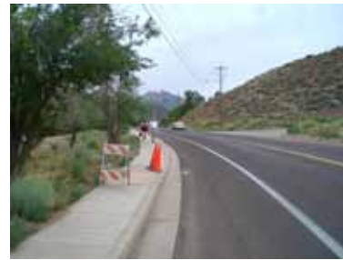
Looking South - D
