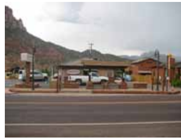
Shuttle Stop - Looking South
