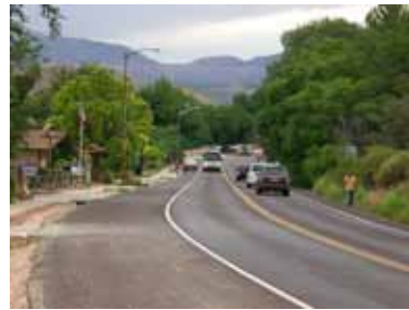
Looking Southwest - C
