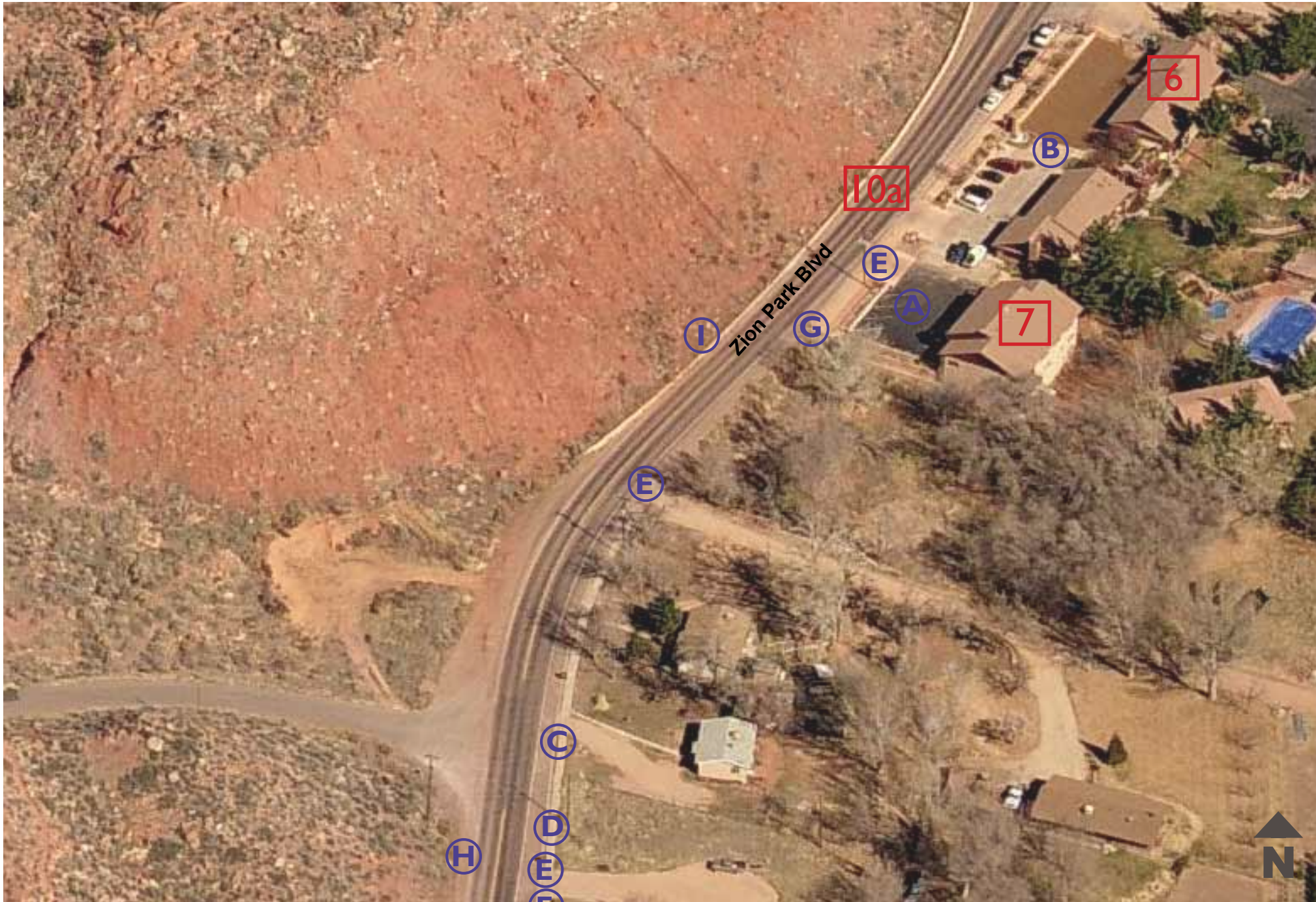
Zion Park Boulevard - 10a On-Street Parking, 7 Tribal Arts, 6 Cliffrose
