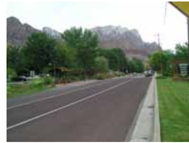
Zion Park Blvd - Looking North
