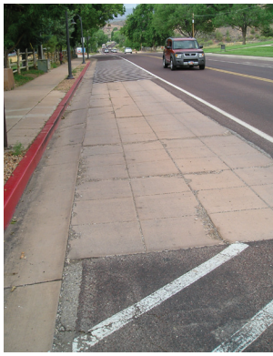
Concrete shuttle pad at Driftwood Lodge
