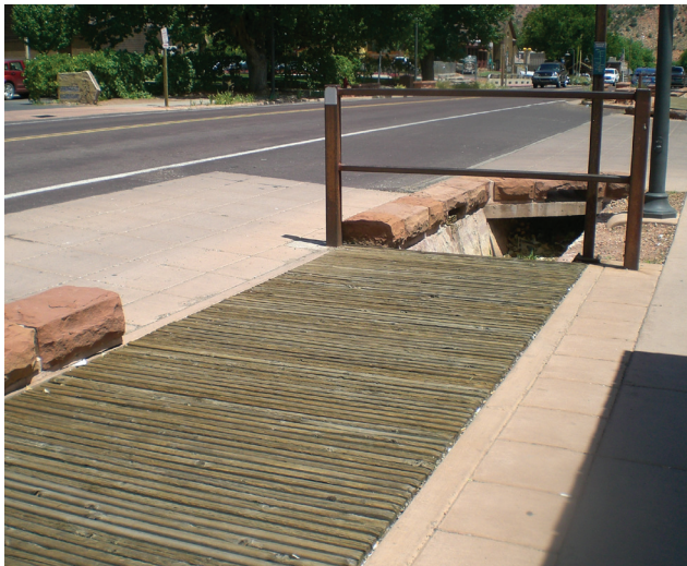
Wood slat platform at Bumbleberry/Zion's Bank shuttle stop platform
