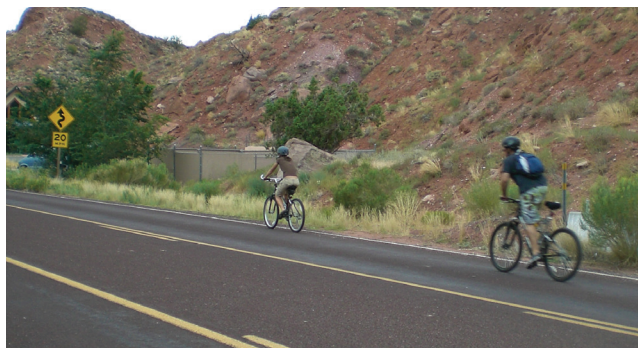
Bicyclists riding in the travel lane at the landslide area
